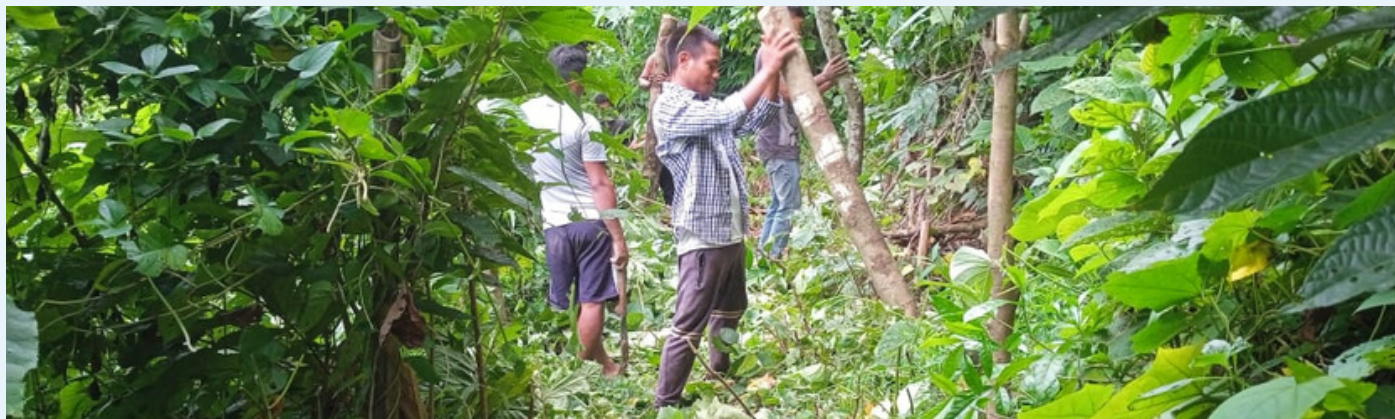
Fencing work at chiringpara village.
