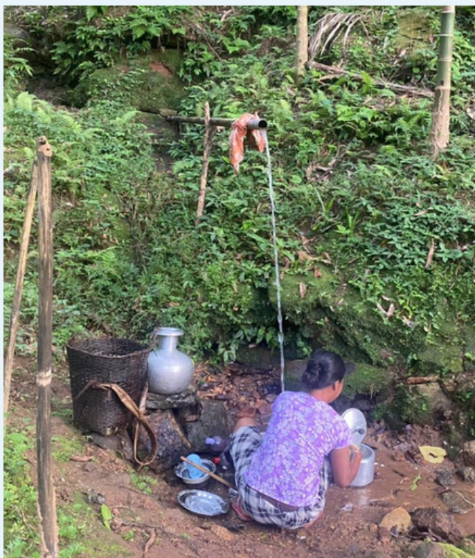
The selected site for the RCC storage tank that will benefit 7 households.
